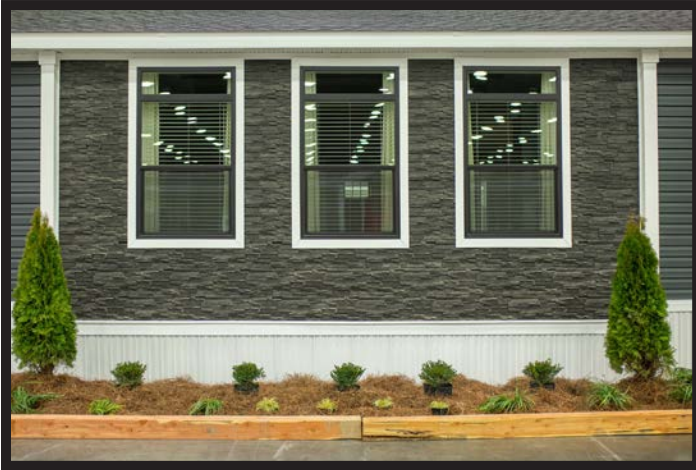
2 Columns w/ Vinyl Rock Accent & Black Windows
