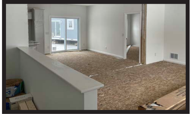
Basement Entry w/ Half Wall & Wood Cap
